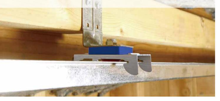
This section describes the elastic sound insulation clamps mounted on plasterboard grooves that support plasterboard, wood, concrete, etc., for wall and ceiling sound insulation (separation coupling).
